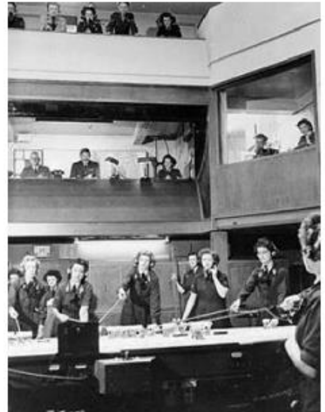
Operation Room at Air Group 10
